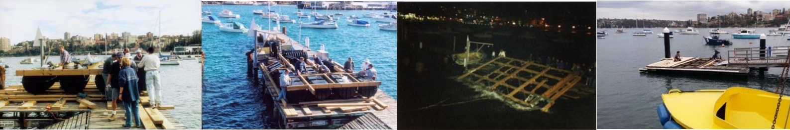
progress images of the pontoon being built
