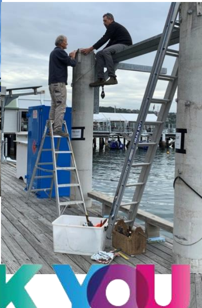
Preparation for the new winches
