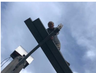
Next job - the spreader bar
